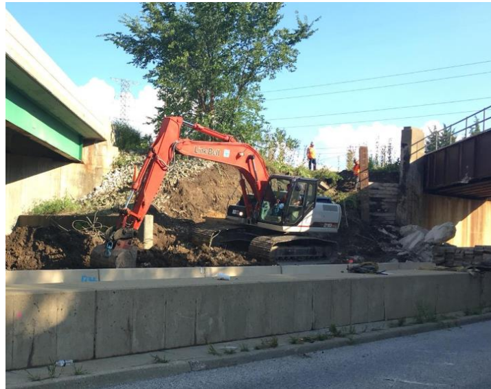
on Sept. 4, 2018, work to remove debris and replace a concrete wall that collapsed along Route 45 between a railroad bridge and the Route 137 overpass. (Lake County Sheriff's Office)
