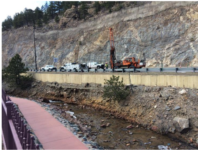
Wall and Slope (rock cut) on ROW and within boundary
