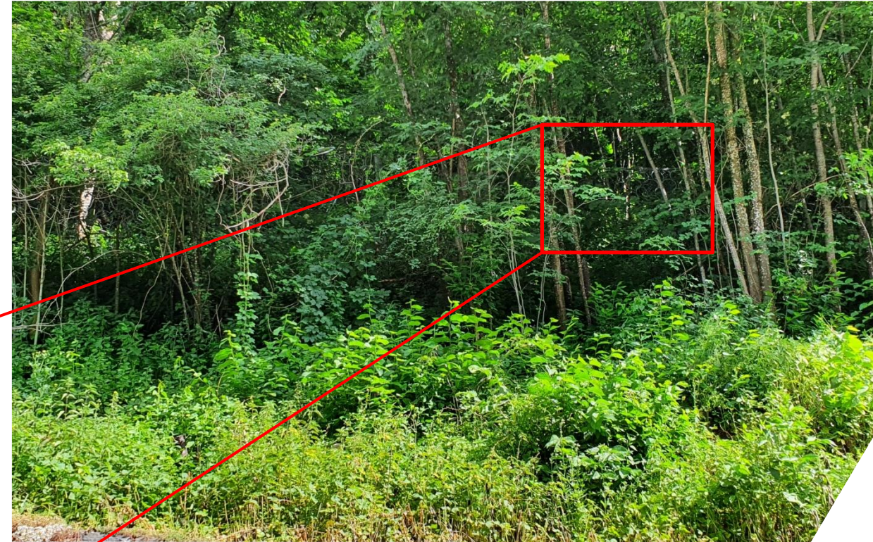
Picture: Visual inspection of a rockfall barrier visible from the road / 21.06.2021
